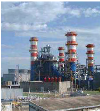
Termocentro power plant conversion project in Colombia
