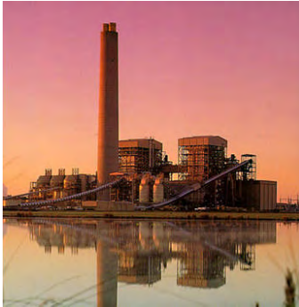
WorleyParsons' full engineering services brought the 540 MW Cross Station Unit 1, one of the few utility baseload plants built in the U.S. during the 1990s, on line six months ahead of schedule.
