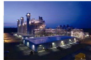
Tenaska Virginia Power Project – DBIA-MAC 2005 Best Project Industrial/Process Sector Over $25 Million, PCIVER Magazine Top Plants
